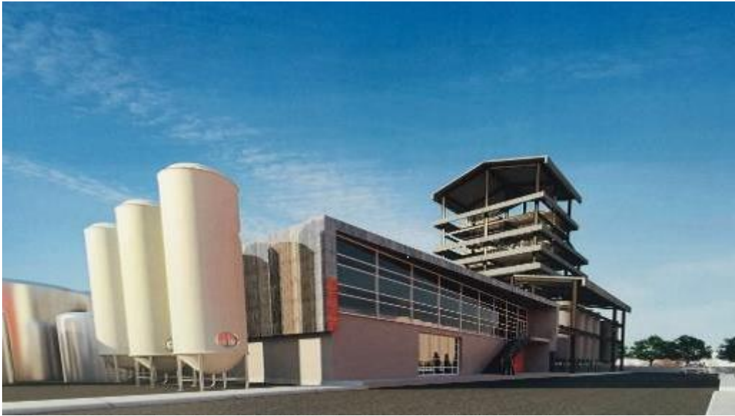
The Western Foods and Packaging margarine manufacturing plant at Serasa
