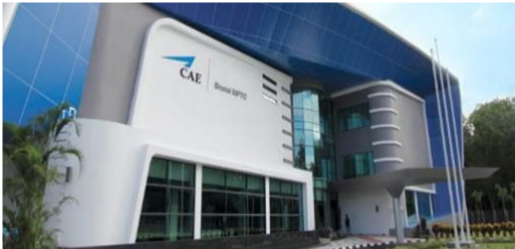
The CAE Multi-Purpose Training Centre at Rimba Digital Junction
