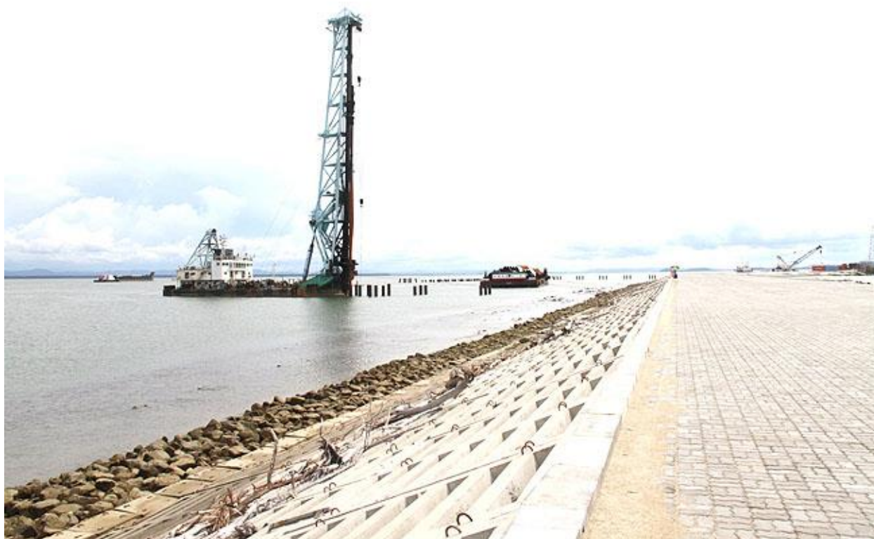
Jetties piling activities at PMB
