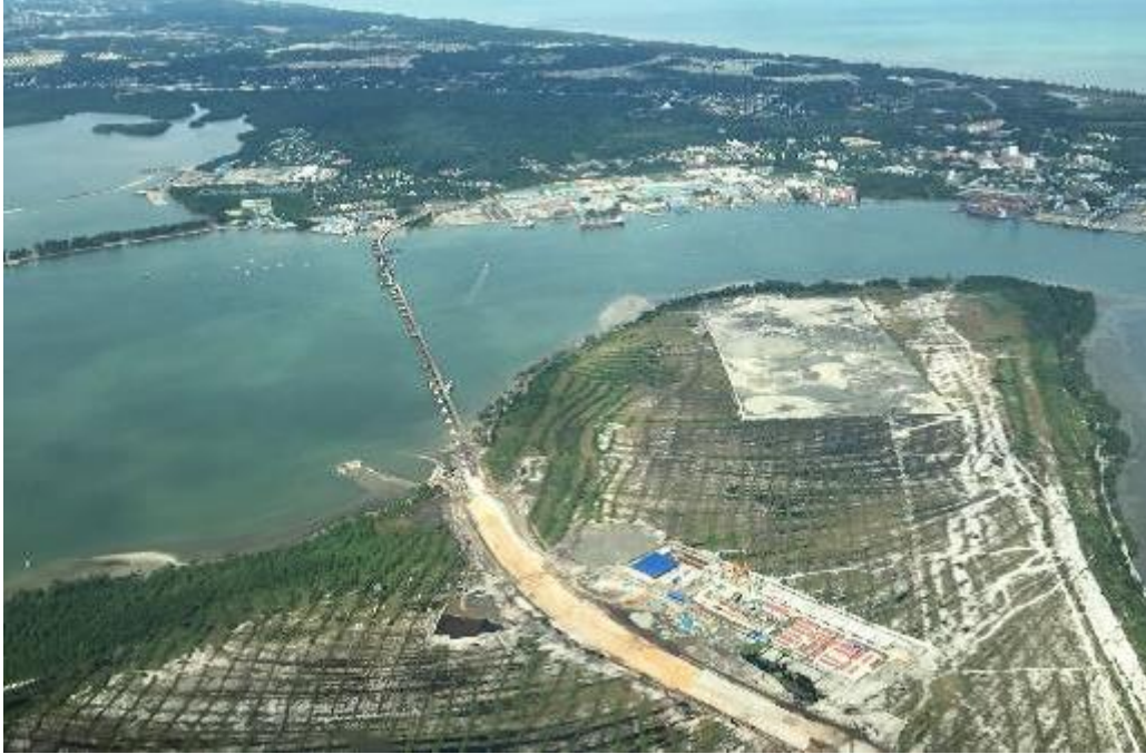
Western Tank Farm & PMB bridge construction
