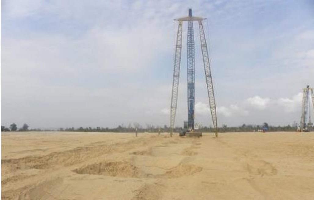
Sandfilling work at PMB
