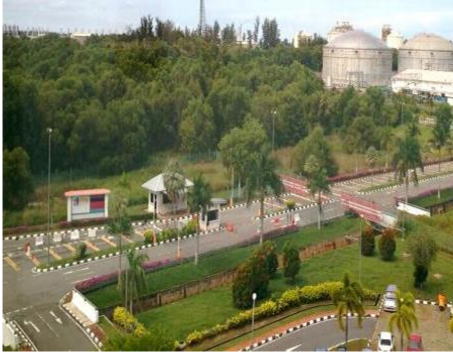
The entrance to the Brunei Methanol Plant
