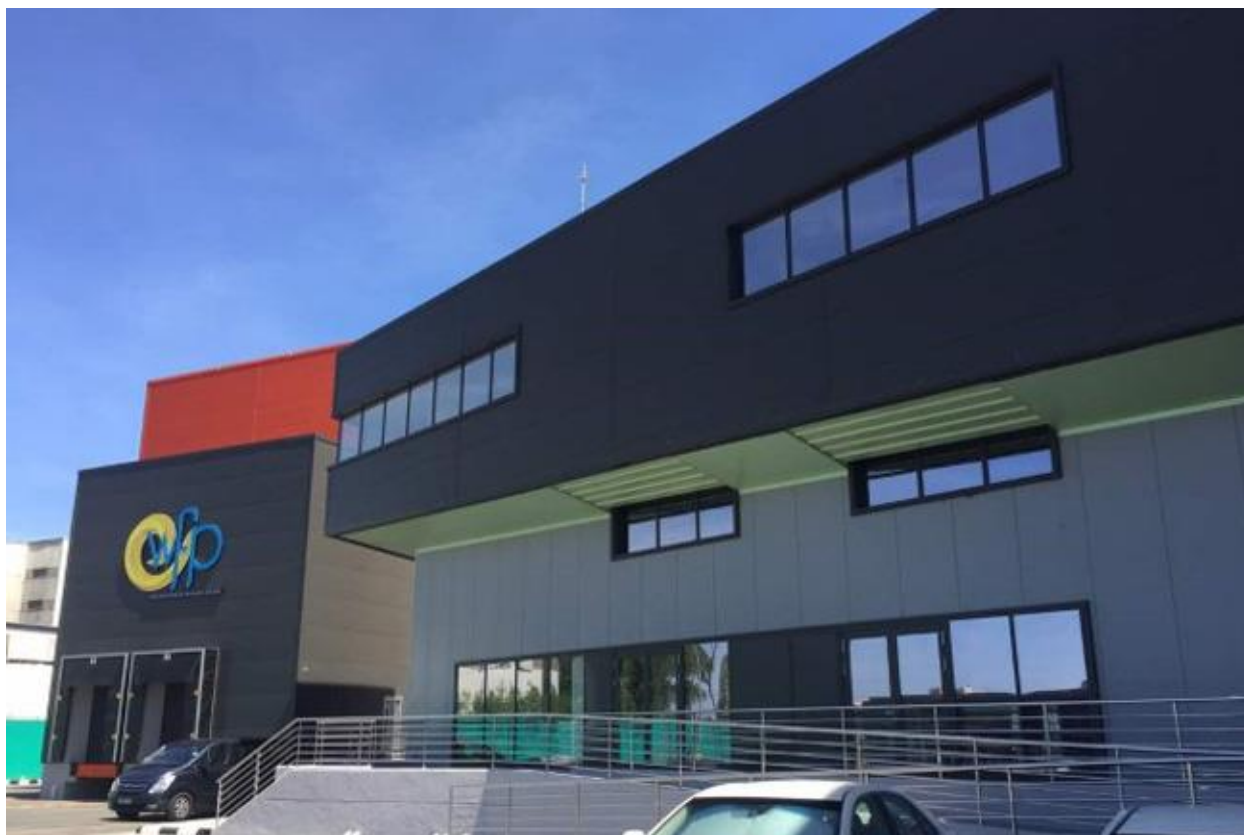
The management building and cold warehouse
